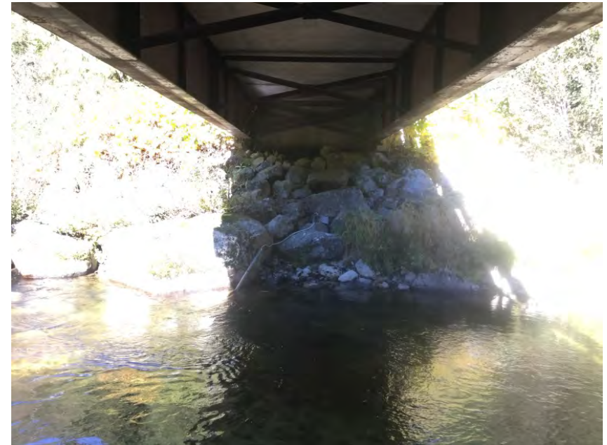
Left Bank Abutment when facing downstream
