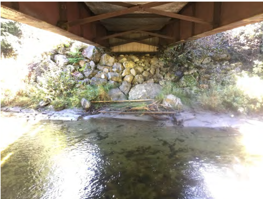
Right Bank Abutment when facing downstream
