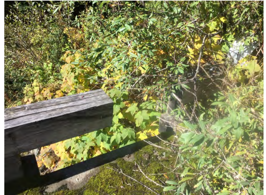
Missing guardrail
